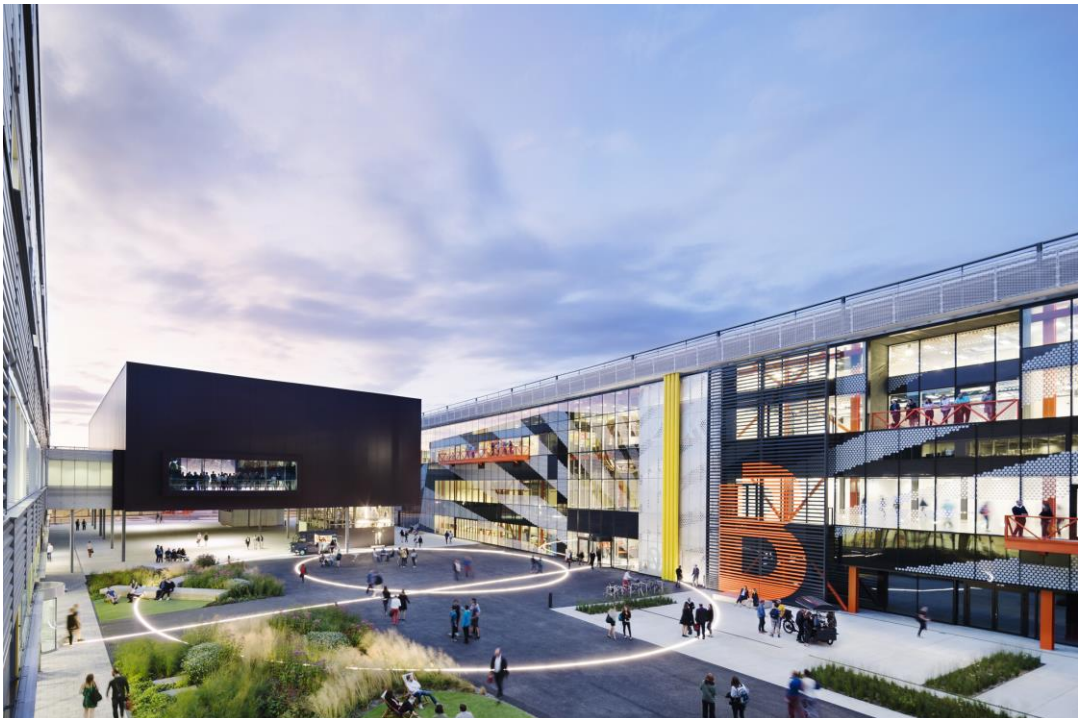
Image courtesy of Here East, London, United Kingdom
